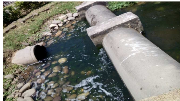
Plate-4 Showing sampling site-4 (Outlet of 27 MLD STP)
