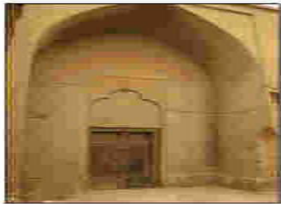
Fig 11: Southeastern entrance (Trading House) in Sigari House in Yazd
