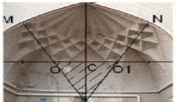
Fig 15: Using blunt cloverleaf latch in southwestern entrance coverage in Sigari House in Yazd (Source: Authors)
