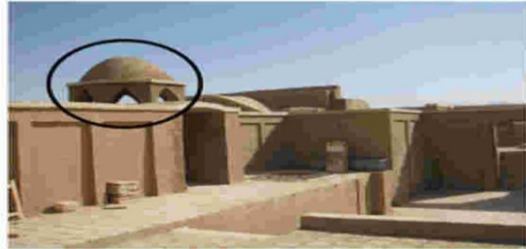
Fig 25: Alcove above porch coverage in trading house entrance (Source: Authors)
