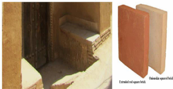
Fig 18: Application of four-squared brick on floor and body of old-sitting platform and forecourt pavement (Source: Authors)
