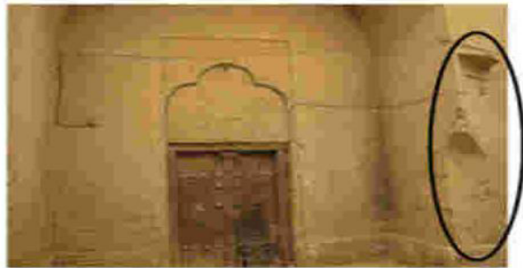
Fig 23: The existing raft for lighting in forecourt wall (Source: Authors)
